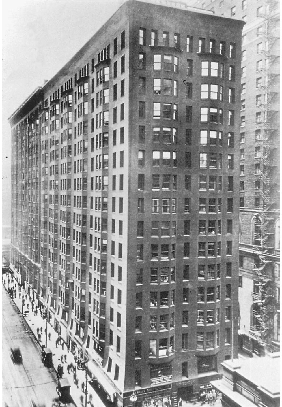
Figure 1-2 The Monadnock Building in Chicago (1891, Burnham and Root architects) was the last unreinforced high-rise masonry building. (Photo courtesy of the School of Architecture Slide Library, the University of Texas at Austin.)
